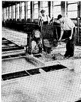
floor fill of perlite concrete can save tons of deadload in multi-story buildings.
