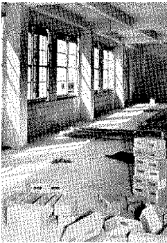
Perlite blocks have 4-hour fire rating in curtain wall construction.
